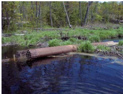
Baffler—before repair
